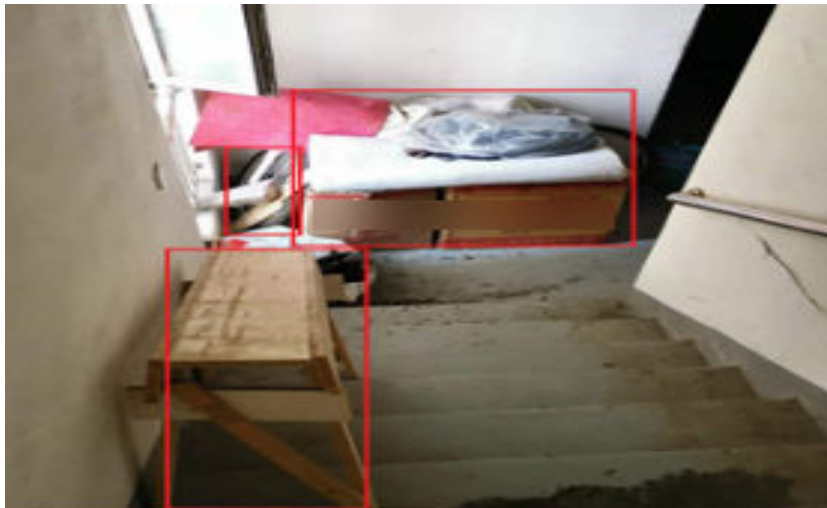
Figure 3-8 Detecting whether fire escapes are obstructed
